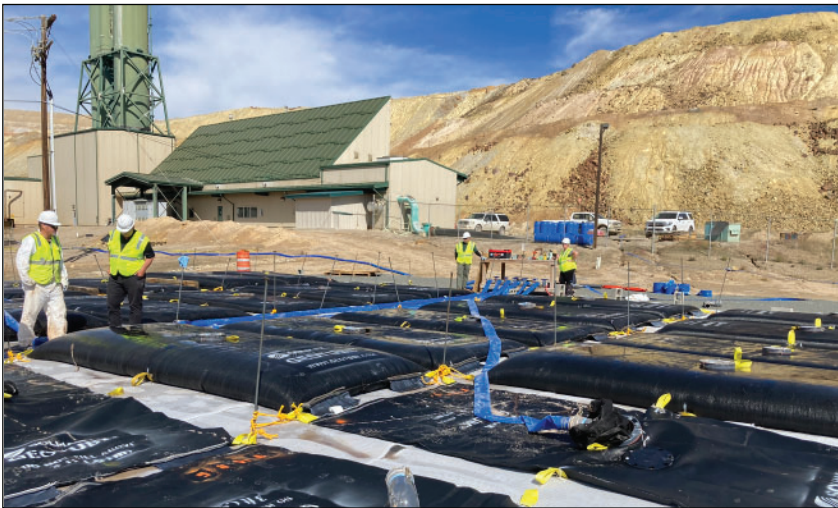
Figure 4. MBMG, MR, and WVU personnel monitoring the filling of sample bags with HPC containing REEs.
