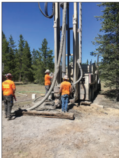
Drilling crew constructing monitoring wells for the NGWMN.
