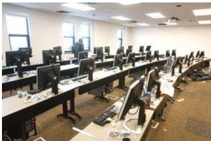
Computers are being installed in preparation for petroleum engineering students who start back to school this Wednesday for the spring semester
