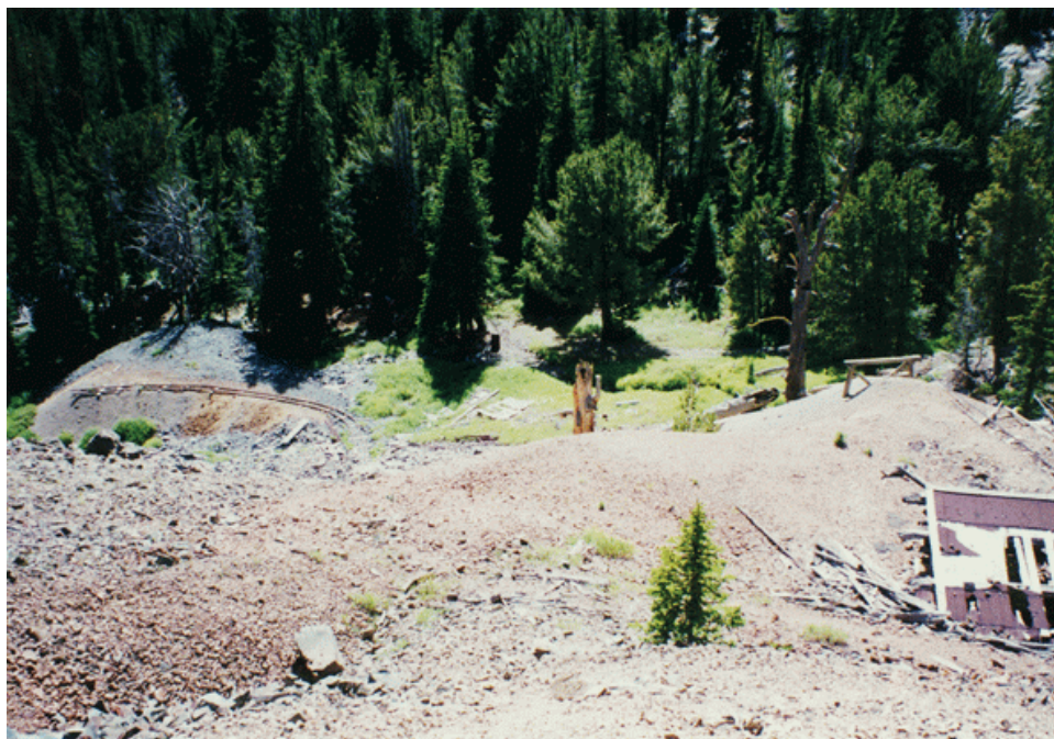
Figure 18A. The stream flowed through the disturbed area of the Skyline mine. The discharge from the middle adit flowed into the stream, which flowed into Leslie Lake.
