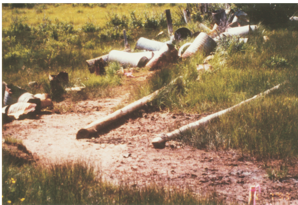
Figure 5B. Cyanide drums were used to construct part of the tailings impoundment.
