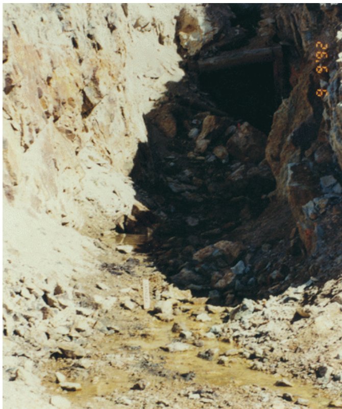
Figure 22C. The Atlantic & Pacific adit discharged acidic water to Park Creek. Waste material was washed into Park Creek when the adit seal blew out.
