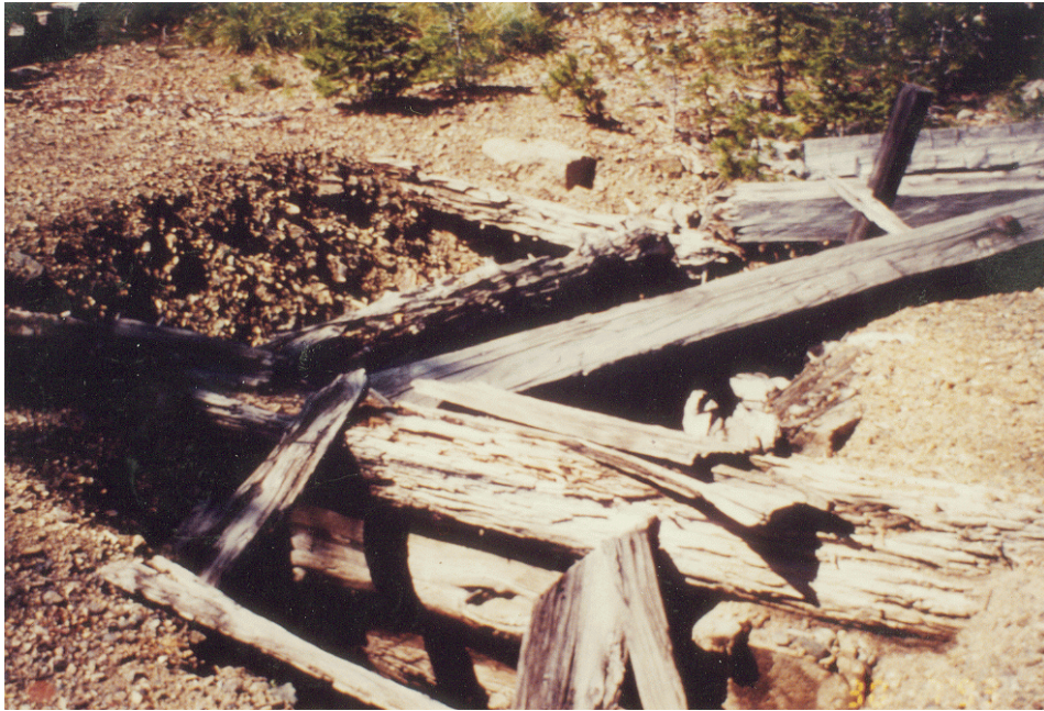
Figure 13A. The west shaft, which was partially flooded and open, is a safety concern at the Leadville mine.
