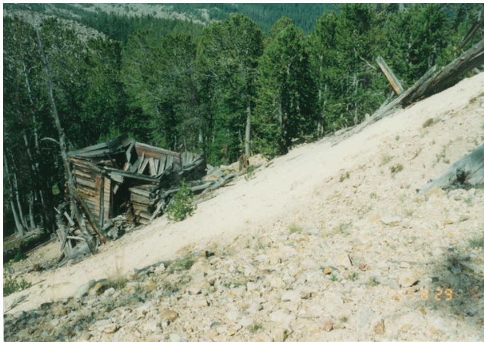
Figure 20B. The waste-rock dump of the Mogullion mine was sparsely vegetated but appeared stable. The ore bin was the only structure observed on the site.
