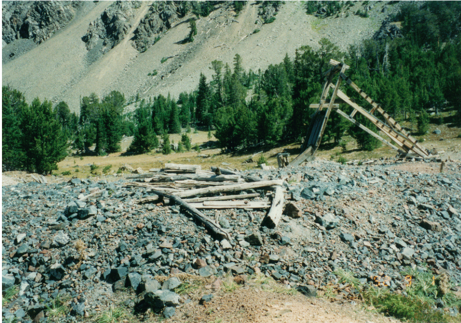
Figure 8A. The Boulder Cobalt mine dump has been reworked. The head frame remains over a flooded shaft.
