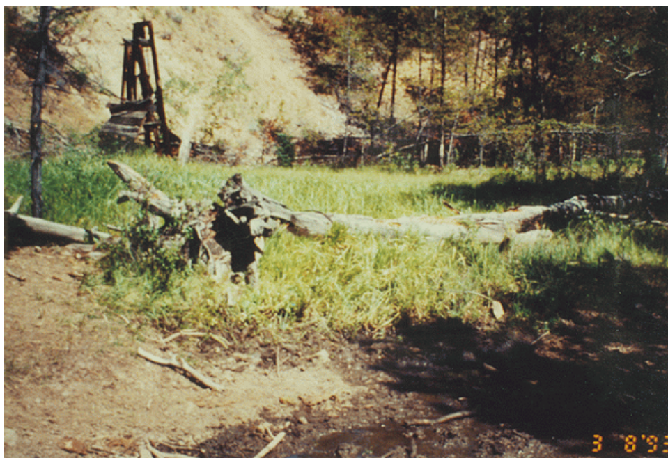
Figure 14A. The discharge from the flooded shaft (beneath the head frame) at the North Boulder Lead mine flowed into a small wetland adjacent to Alta Gulch.
