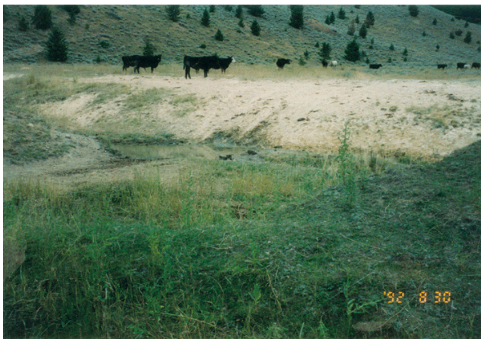
Figure 22B. The tailings impoundment on Park Creek below the Atlantic & Pacific and Viking–Western Pacific development has been eroded by Park Creek.
