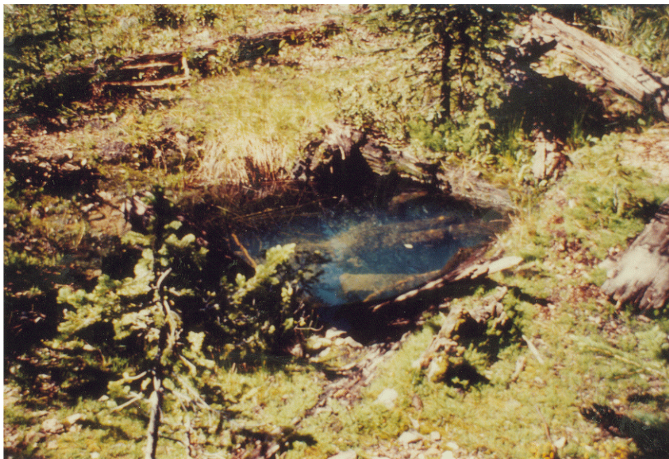
Figure 13B. The middle shaft was open and flooded to the surface; a discharge probably occurs in periods of runoff.
