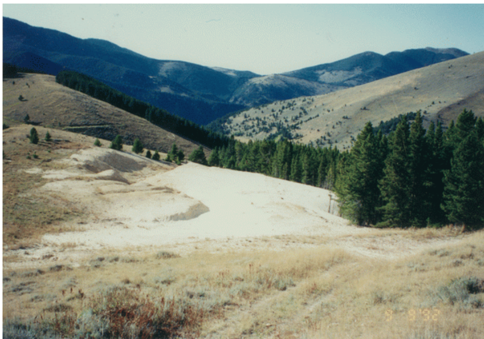
Figure 22A. The tailings of the Atlantic & Pacific are subject to water and wind erosion, as well as small-scale mass wasting.
