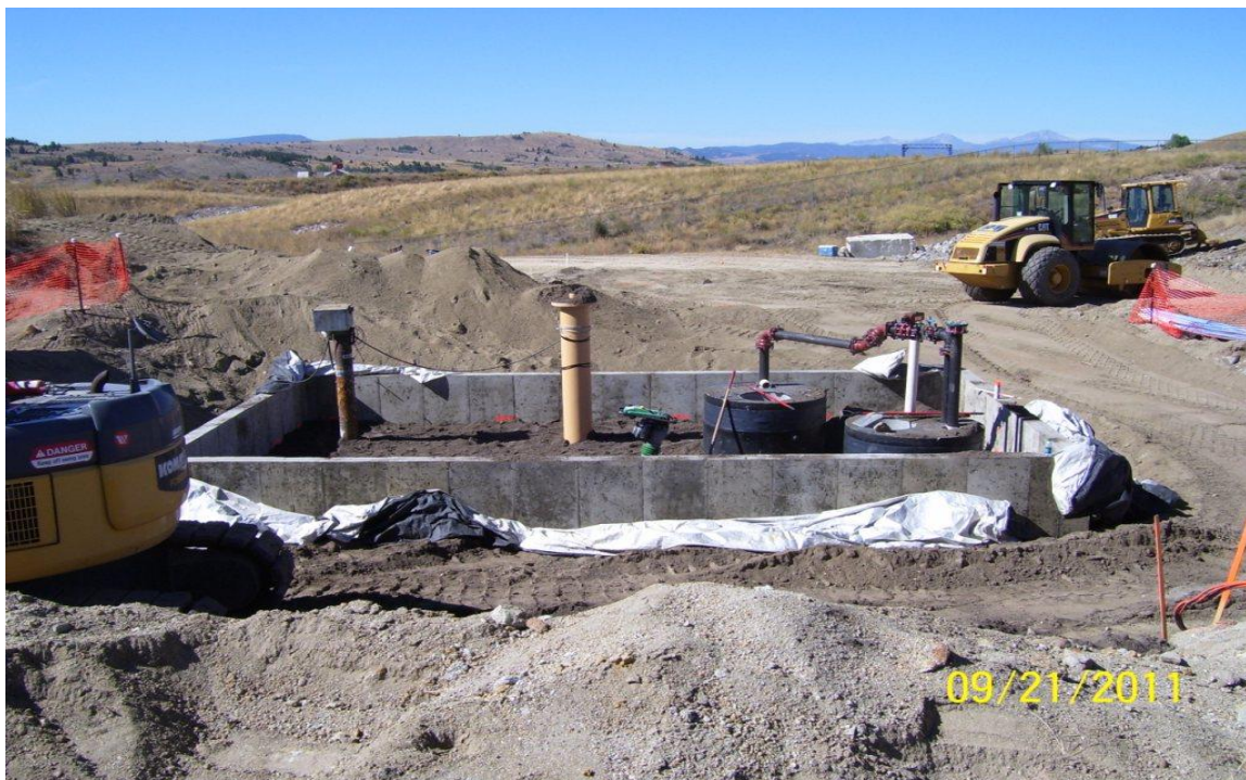
Figure 3-4. West Camp construction activities showing new pump station foundation and infrastructure improvements surrounding pumping well and discharge line.
