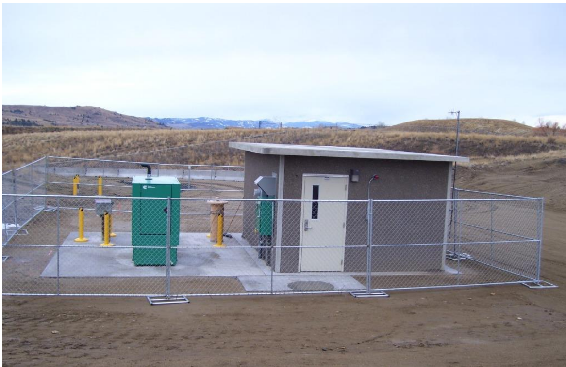
Figure 3-4. West Camp construction activities showing new pump station foundation and infrastructure improvements surrounding pumping well and discharge line.
