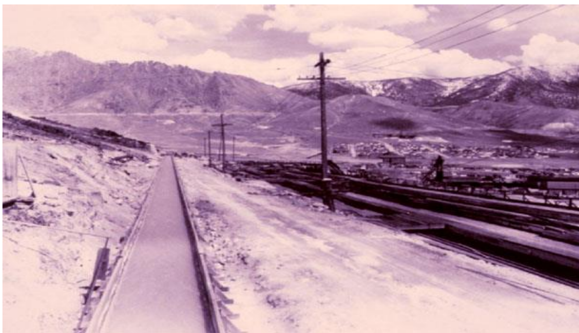
Figure 1-3. Flume conveying water pumped from Butte underground mines to precipitation plant. (Photo courtesy World Museum of Mining, Butte, MT.)
