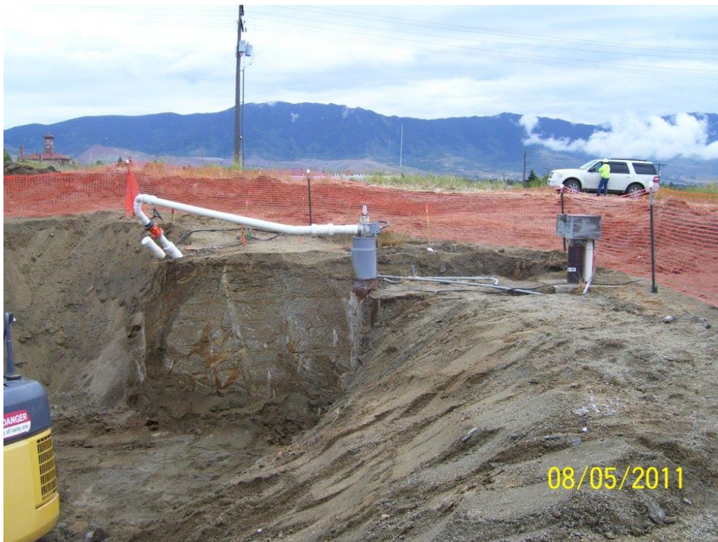
Figure 3-3. West Camp pumping well, discharge line, and monitoring well exposed during 2011 construction activities.
