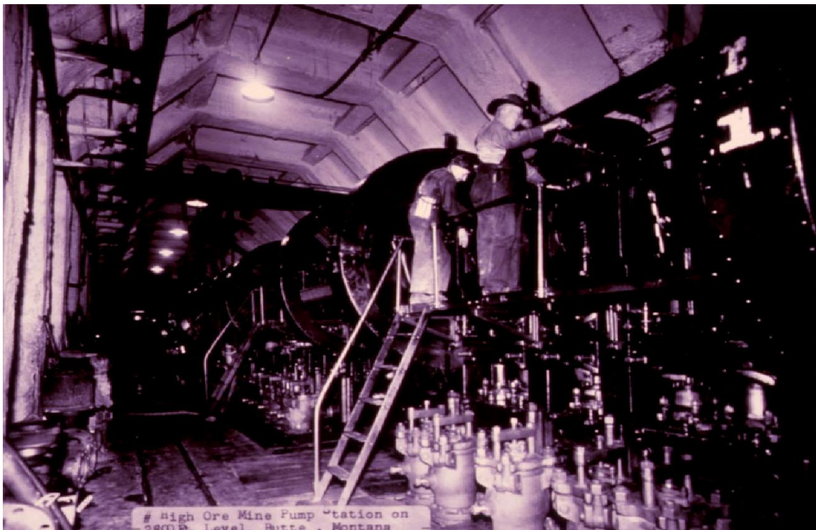
Figure 1-1. High Ore Mine pump station, 2800-ft level. (Photo courtesy World Museum of Mining, Butte, MT.)
