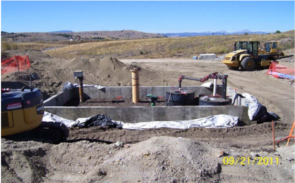
Figure 3-4. West Camp construction activities showing new pump station foundation and infrastructure improvements surrounding pumping well and discharge line.
