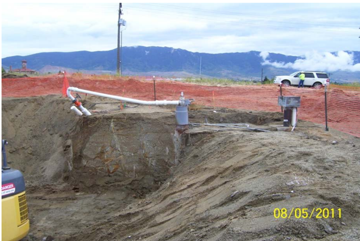
Figure 3-3. West Camp pumping well, discharge line, and monitoring well exposed during 2011 construction activities.
