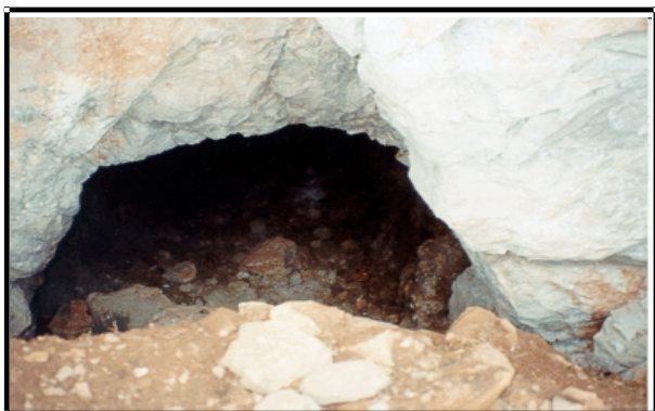
Adit partially blocked by collapse of hill slope.
