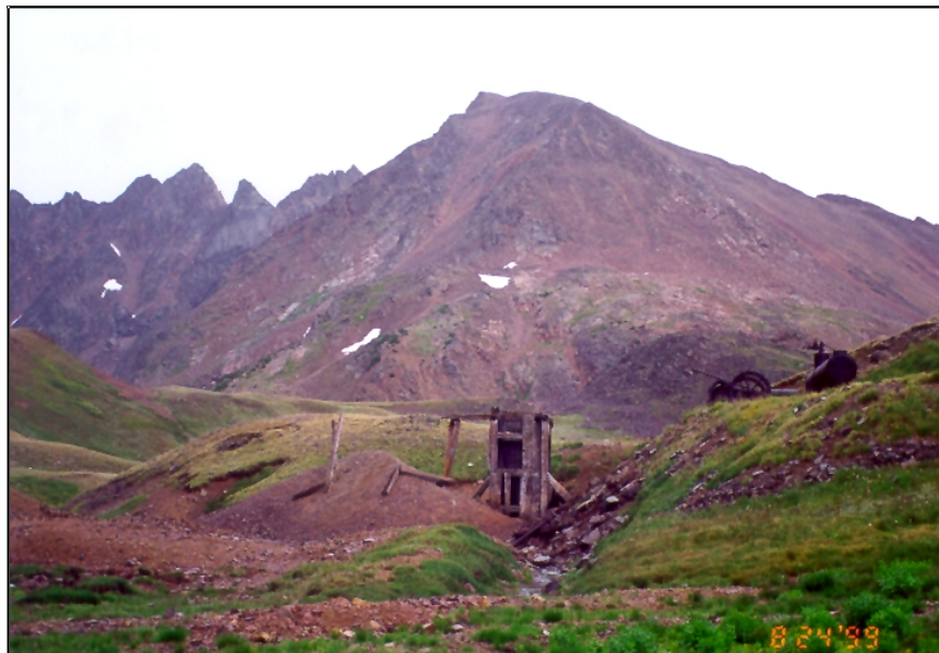
Figure 5b. The private Copper King shaft is flooded and was discharging into Goose Creek.
