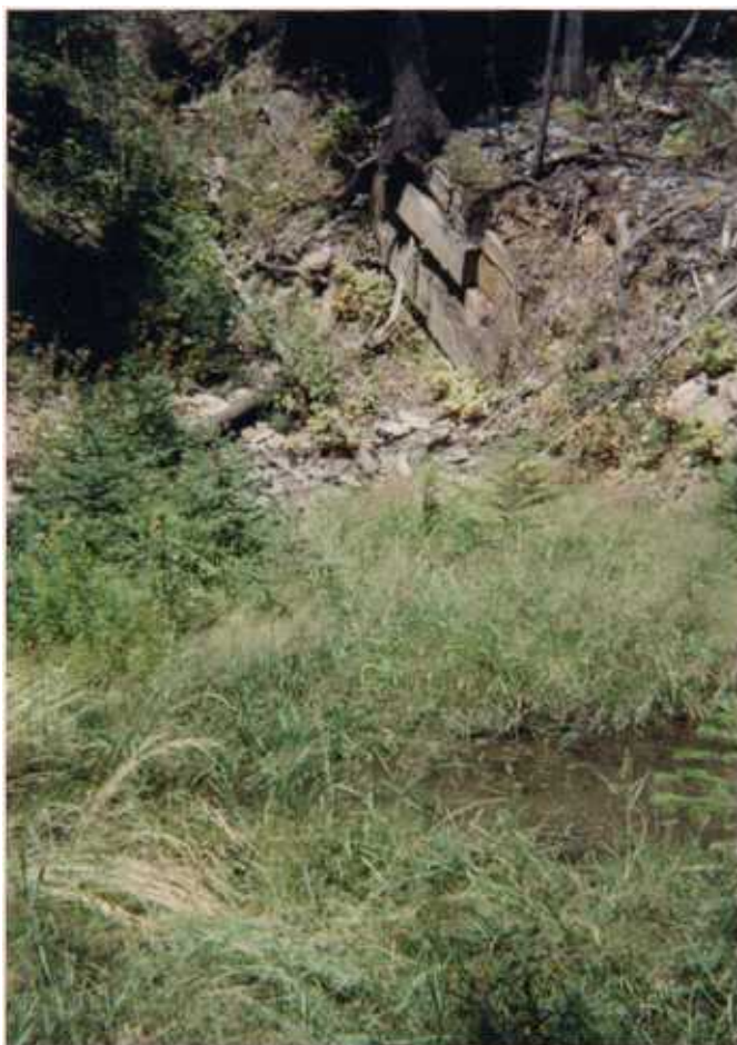
Figure 21a. A seep emerged from the collapsed adit portal at the Copper Reward, flowed approximately 20 feet where it formed a small pool on the waste dump. It then infiltrated the dump.
