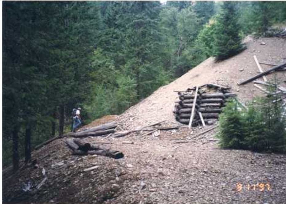
Figure 10b. The Broken Hill waste dump was steep and largely unvegetated with the slope reflecting the steep topography surrounding the site.
