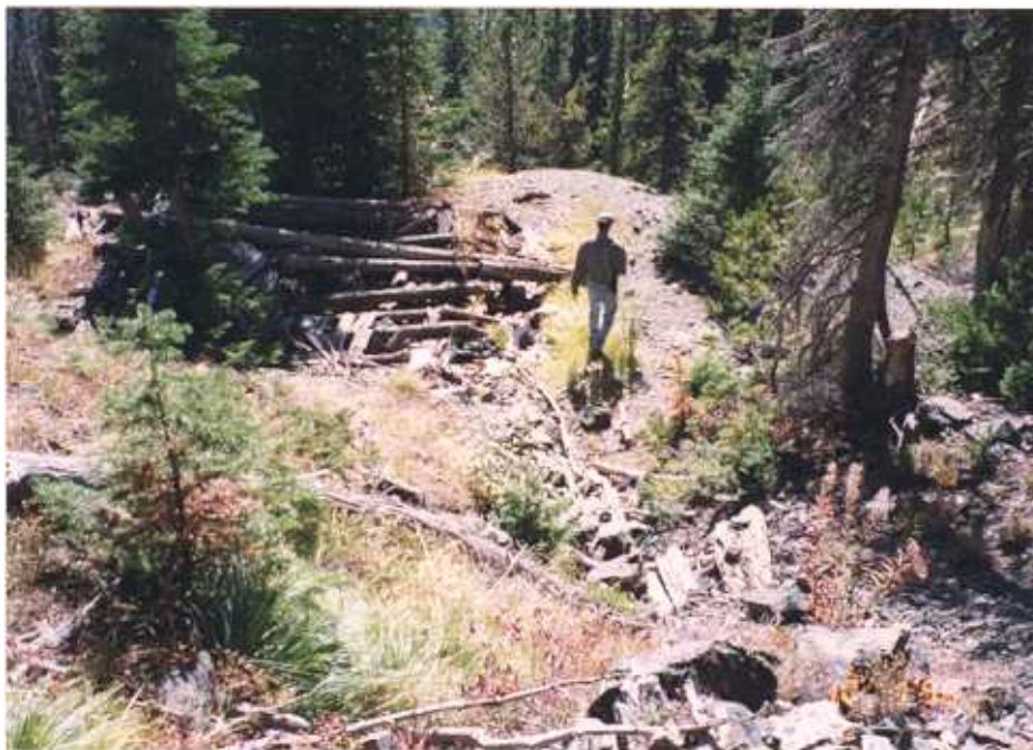
Figure 15b. Looking down from the talus and upper caved adit at the Independence, the adit can be distinguished by the green grass in front of the geologist.
