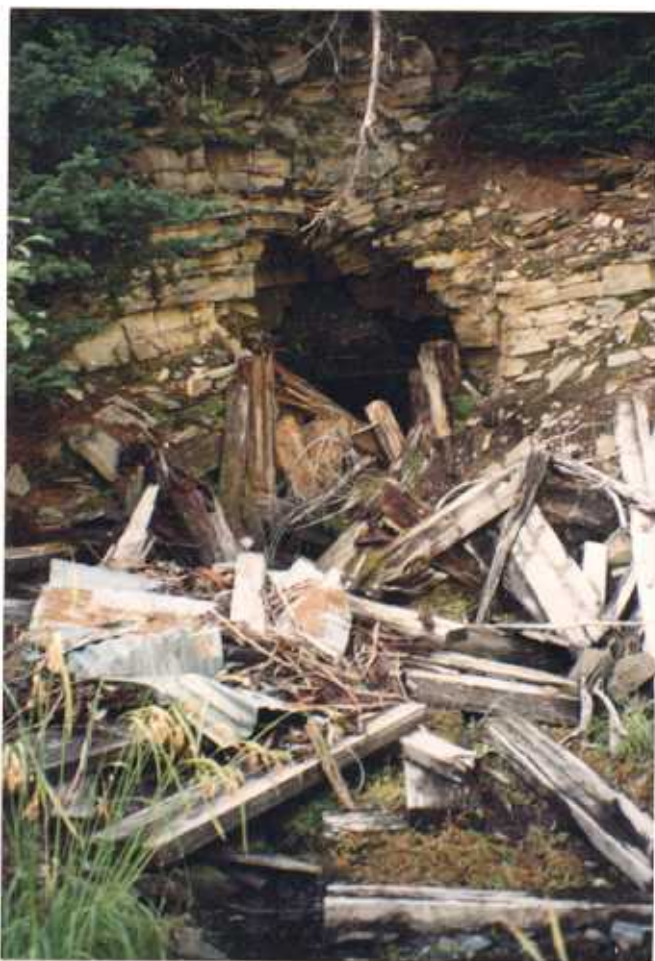
Figure 4a. The Montana Tunnel at the Jack Waite is open and had a small discharge of water that completely infiltrated into the waste dump.
