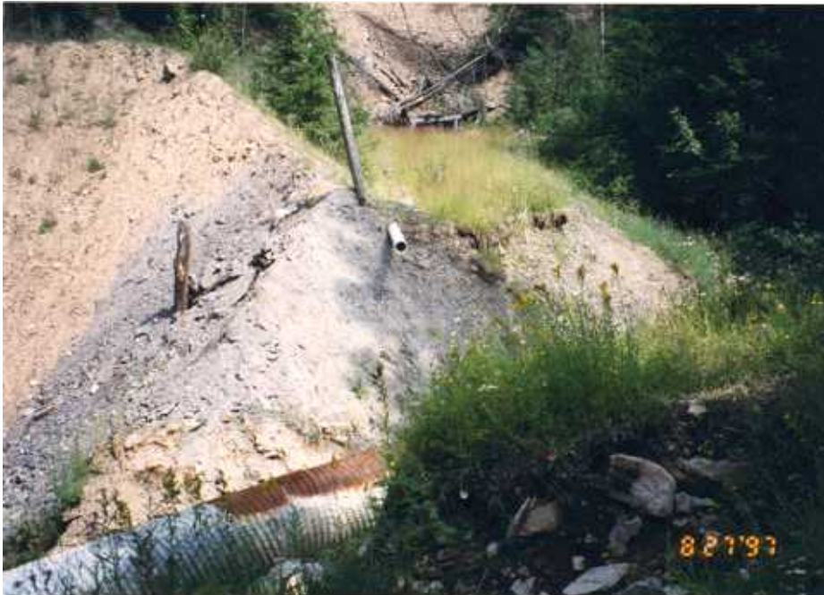
Figure 6b. Granite Creek (at low flow) has cut the waste dump at the Ambassador, resulting in an easily erodible face. The partly open adit lies in upper center of the photo.
