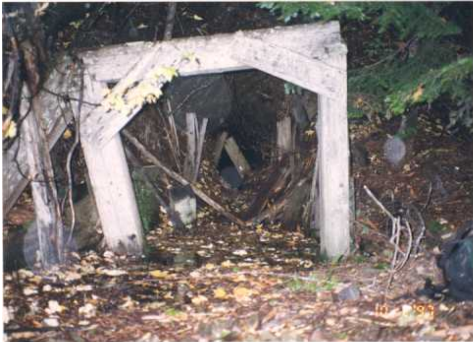
Figure 29a. The open adit at the Giant Sunrise held standing water but none was flowing at the surface to the active drainage.
