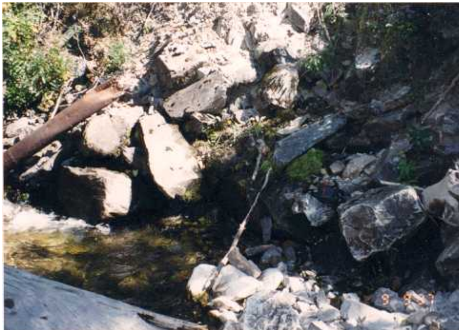
Figure 7b. The discharge from the Heidelberg infiltrated into the waste dump and discharged at the toe. The discharge emerges just below the camera case used for scale.
