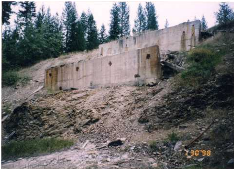
Figure 23b. The foundation of the mill at the Cherry Creek site posed a safety threat because of erosion at the footings.
