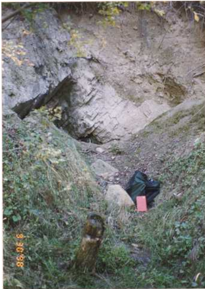
Figure 12a. The adit near Rock Lake was predominantly caved with a small rate discharge flowing from the caved portal.
