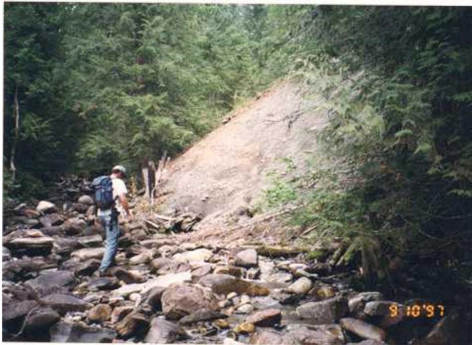
Figure 11a. The waste dump at the Blue Creek mine would be in contact with the creek during high water flow.
