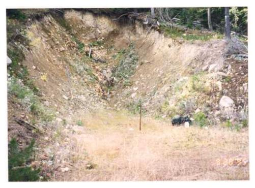
Figure 10a. The collapsed adit of the Viking mine discharged about 0.5 gpm. No other discharges were observed on or near the site.
