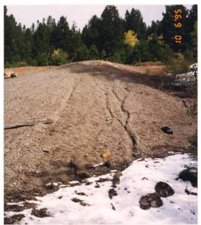
Figure 15a. Erosional rills marked several large waste-rock dumps on a steep hillside at the Kimball mine.
