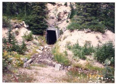
Figure 29b. Five-gpm discharge emerged from the lower Copper Camp adit that was caved beyond the lagging.
