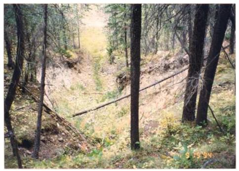
Figure 21b. Looking NW along the collapsed adit at the Bumble Bee with the small greenish discharge channel visible in the center of the photo.
