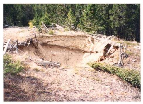
Figure 21a. One of two dry, collapsed shafts found at the Bumble Bee/Morning Star.
