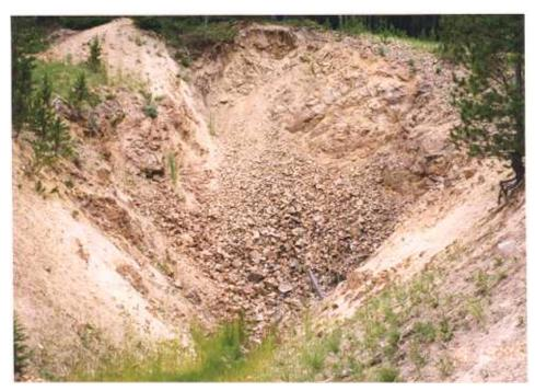
Figure 7a. The collapsed adit at the Hope mine discharged about 1 gpm. The highwall was steep but generally stable.
