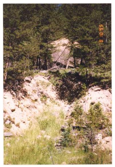
Figure 8a. The collapsed adit of the Hub Camp mine discharged about 1.5 gpm, which infiltrated the ground within 100 feet of its origin.
