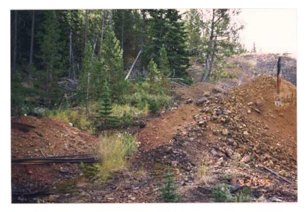
Figure 13a. The lower, caved adit of the Monarch mine was discharging a small amount of water on to the lower waste-rock dump. The adit lies in the trees just left of center.
