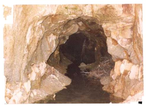
Figure 4a. The adit of the North Ontario mine remained open at least 40 feet from the surface. The tunnel was partially flooded and discharged water on to the dump.
