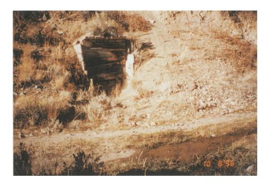
Figure 2.12 The condition of the Paradise Claim's adit is unknown because the portal is closed with a wood door that can not be opened.
