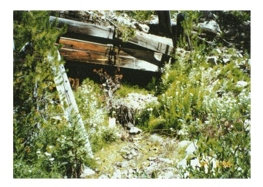
Figure 3.12 A slight mass movement of earth has occurred upslope from the collapsed adit south of the open pit.
