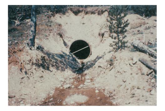
Figure 3.53 A 5-gpm discharge flows from the collapsed adit at the Queen of the Hills mine.
