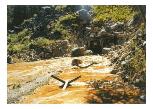
**Figure 3.24** The discharge from the Elkhorn mine main adit splits into two channels; when the site was visited in September 1996, the flow was estimated at 150 gpm.
