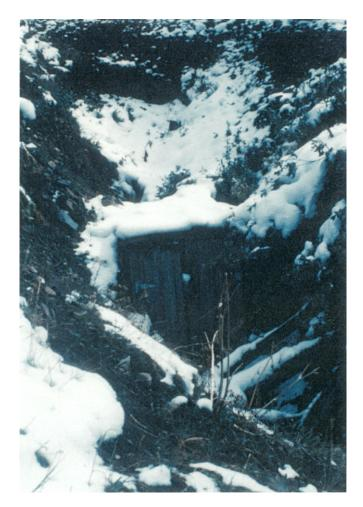
**Figure 4.6** The discharge from the lower adit eventually joins the discharge from upper adit. The combined flow rate of the discharges is about 5 gpm.
