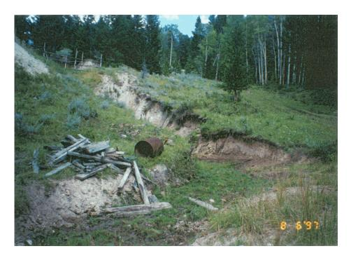
Figure 3.18 The collapsed adit has a small, probably seasonal discharge, that flows across a flat area and soaks into the ground.
