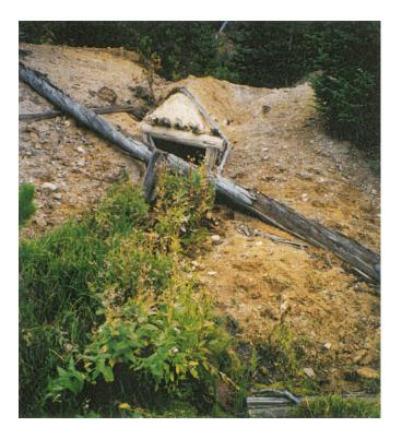
**Figure 2.8** The collapsed adit with a discharge at the Copper Queen mine was sampled downstream.
