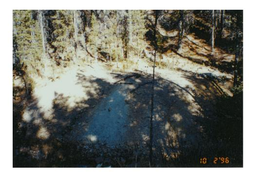
Figure 3.5 The toe of the larger waste-rock dump is in contact with Elkhorn Creek.
