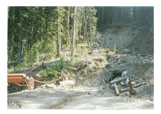
**Figure 4.29** The lower adit has a small discharge that flows across the waste-rock dump before sinking into the ground. An old truck, a trailer, and some other equipment are located near the portal.
