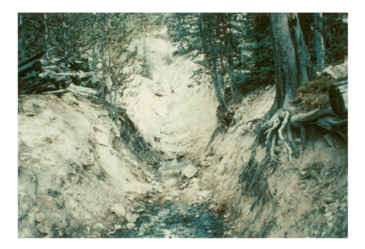
Figure 3.47 A small discharge flows from the collapsed portal of the main lower adit.
