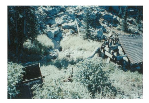
Figure 3.44 The partially collapsed adit at the Jahnke mine has a large, clear discharge.
