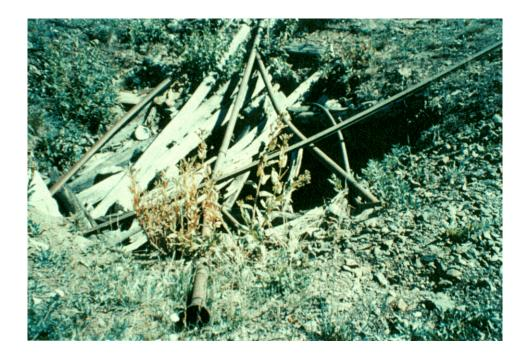
**Figure 4.10** The poorly marked S-1 shaft is a safety concern because it is located next to a heavily used ATV trail.
