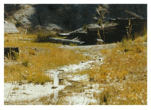
Figure 3.27 A small discharge flowed from the collapsed adit and soaked into the ground.
