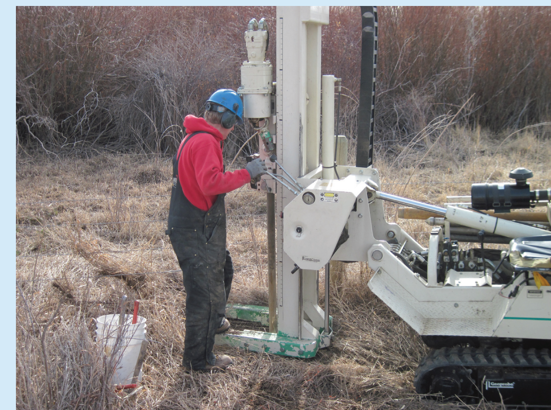
Installing a piezometer adjacent to Sevenmile Creek
