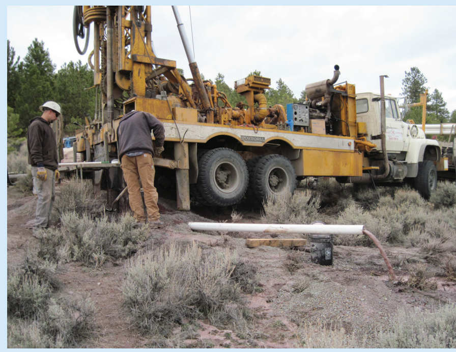
Installing a well at the Helena Valley Fault Site
