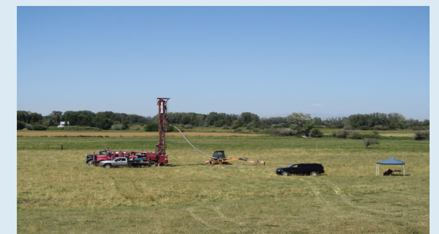
Monitoring Well Drilling
